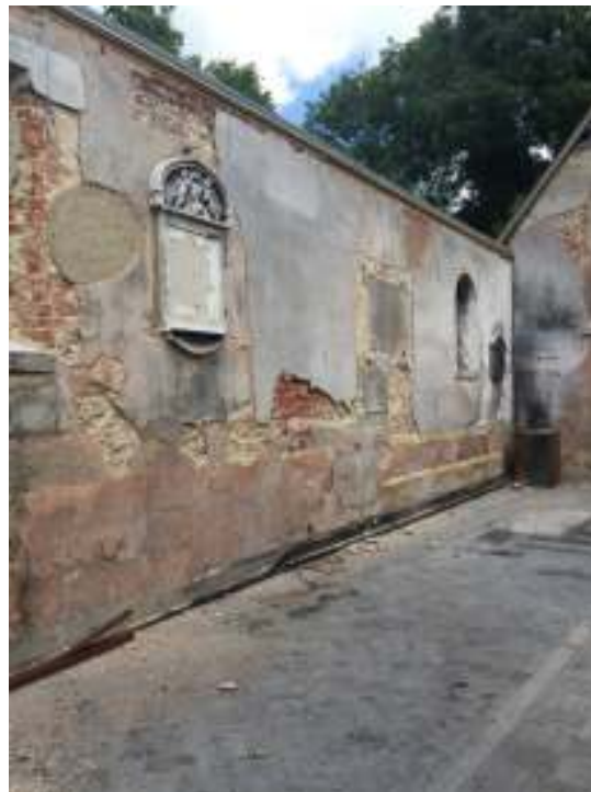
Photograph of Eastern Section of North Wall
