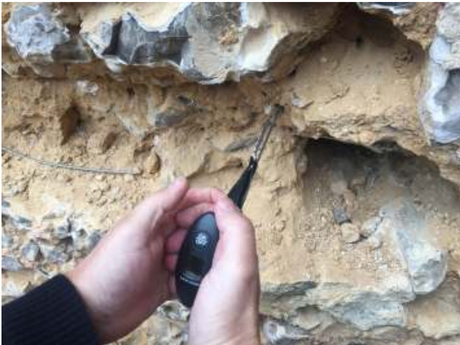
Photograph of Wire Tie and Pull Out Test
