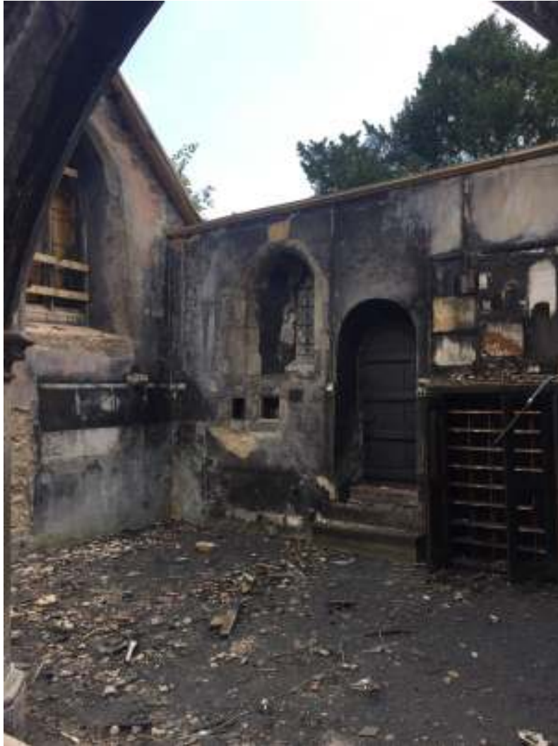
View Of The East Section of the South Wall
