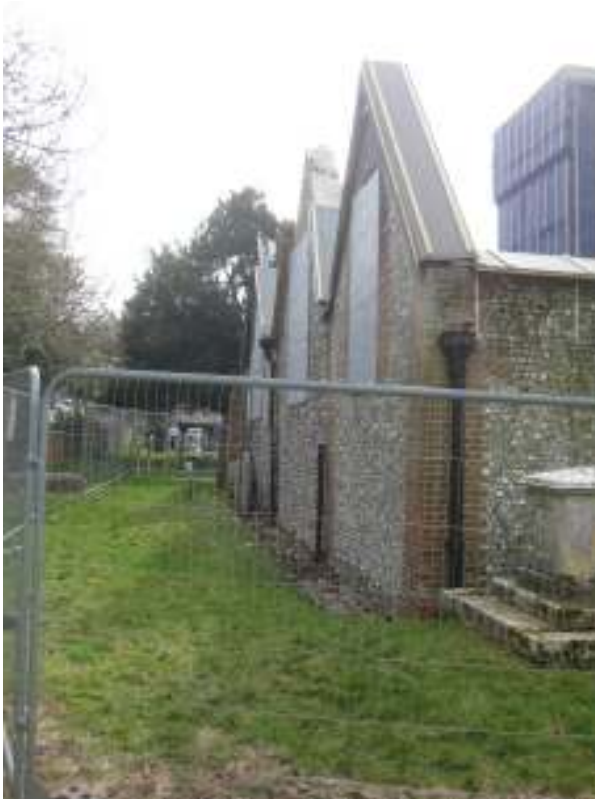
Photograph Of External Face of Eastern Vestry Wall
