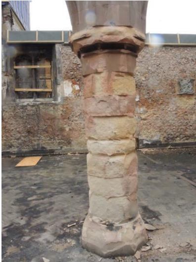
An arcade pillar
